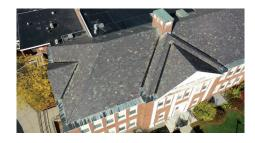
Portions of the slate roof will be replaced and flashing installed to repair leaks.
